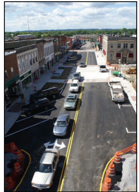
North Water re-opens with new sidewalks, plaza areas, brick crosswalks, additional parking and landscape islands.
