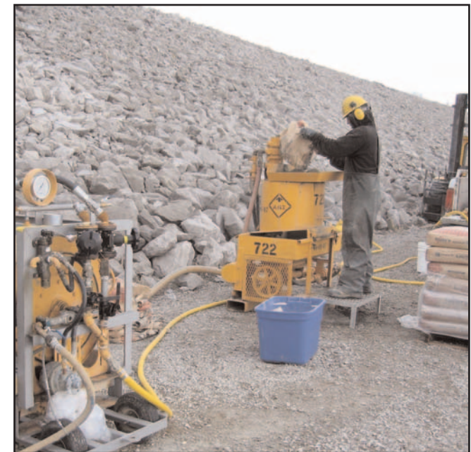
January 2007 grouting operation at the earthen embankment
